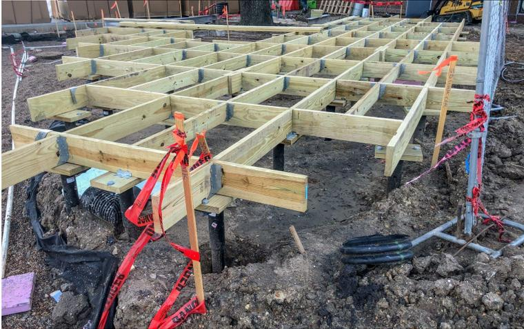
An arbor was called in to locate the root systems of the trees. The roots made the lay-out of the helical piles challenging but Ram Jack was able to deliver with no damage to either tree.
