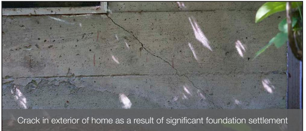
Crack in exterior of home as a result of significant foundation settlement
