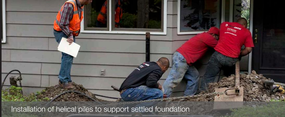
Installation of helical piles to support settled foundation
