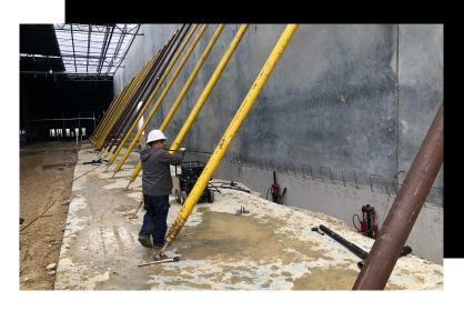
It was quickly determined that some of the existing concrete piers were under designed to support the structural loads of most of the tilt wall panels and the mezzanine. Alpha Testing had worked with Ram Jack and Fortified Engineering Solutions on a similar project so recommended them on this one.
