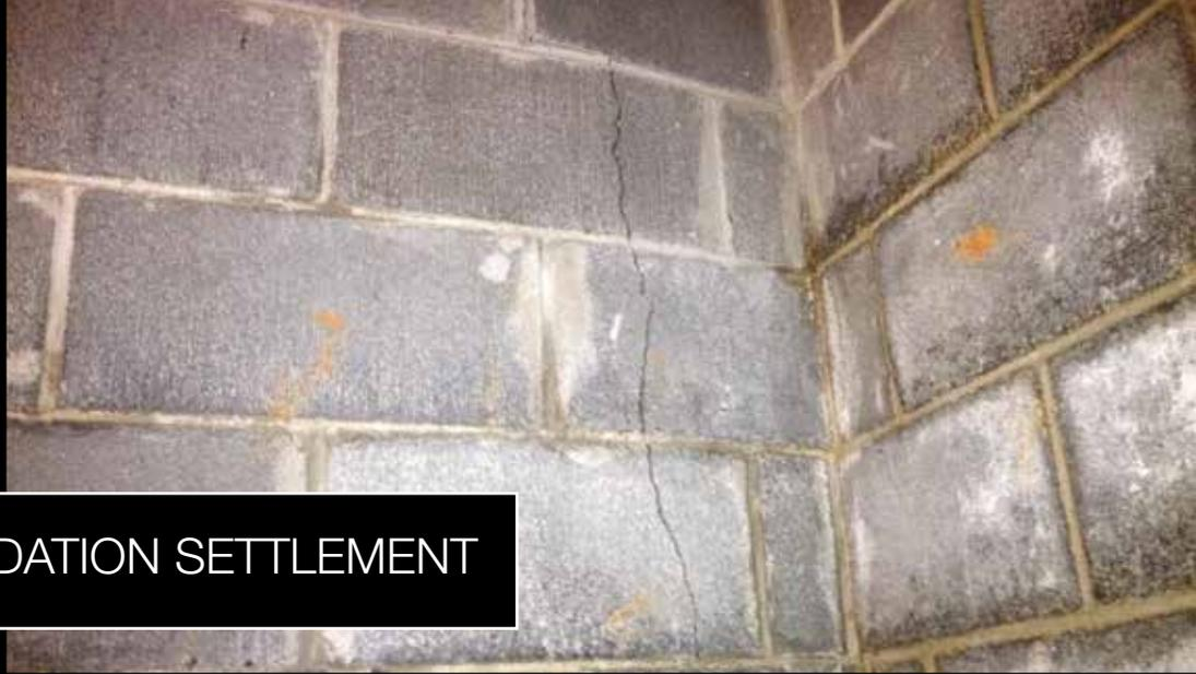
Foundation settlement can lead to a wide array of problems for any home. Whether it's sagging walls with cracked bricks or a sinking driveway with an uneven slope, the damage can be severe and overwhelming. The fact is that when a foundation settles, it doesn't discriminate, wreaking havoc on whatever it supports.
