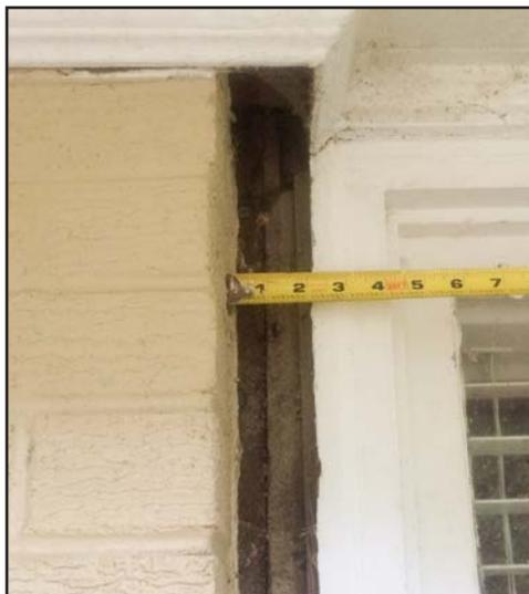
BEFORE: Foundation settlement caused 2-inch gap
