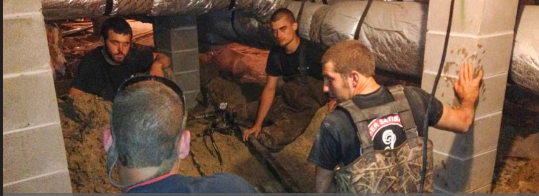
Crew installs helical piles in crawl space
