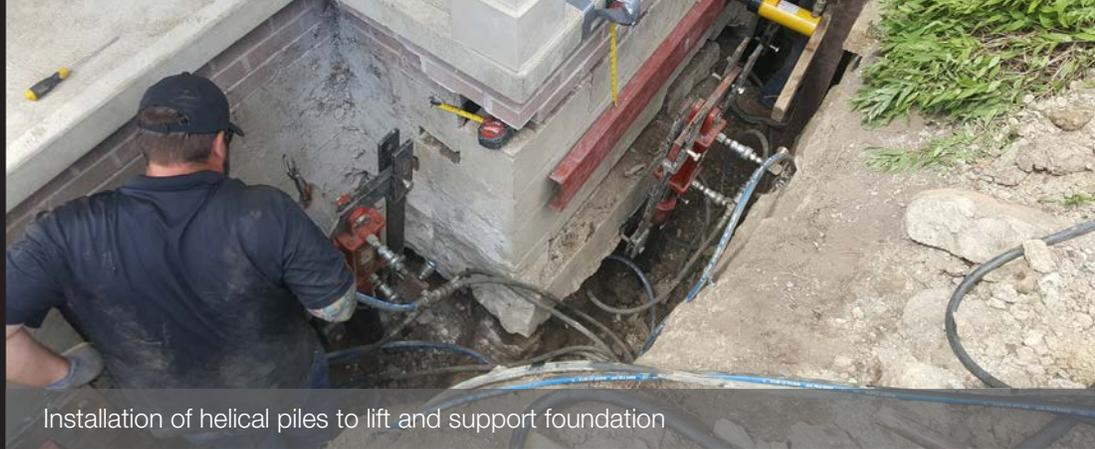
Installation of helical piles to lift and support foundation
