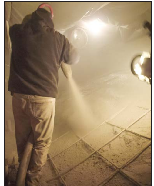
Shotcrete being sprayed after helical tie-backs were installed
