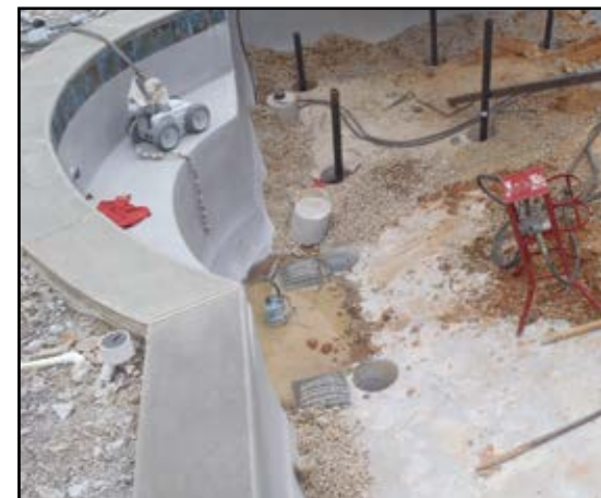
BELOW: underpinning the pool area
