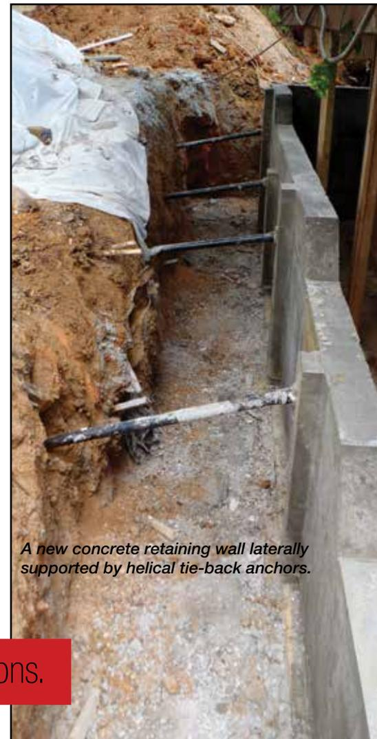
*A new concrete retaining wall laterally supported by helical tie-back anchors.*
