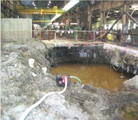
**Situation:** The project consisted of an existing manufacturing facility requiring the installation of a 25'-0" deep precast concrete pit on the interior of the building. The opening of the excavation through the floor slab was approximately 30'-0" x 30'-0" and adjacent to a building column supporting a 133 kip load. Another obstacle encountered was the water table was 12'-0" below finished floor requiring the dewatering of the lower 13'-0" of the excavation.
