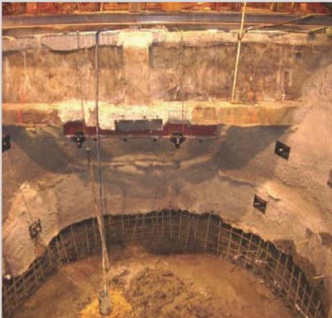
**Solution:** The Larson Engineering, Inc., on the owners behalf, contacted Ram Jack of Illinois (owner: John Walsh) for their expertise in underpinning the undermined column and also provide the shoring and dewatering required to safely excavate and install the 25'-0" precast concrete pit. Ram Jack of Illinois worked with the engineer of record to develop an underpinning and shoring plan.
