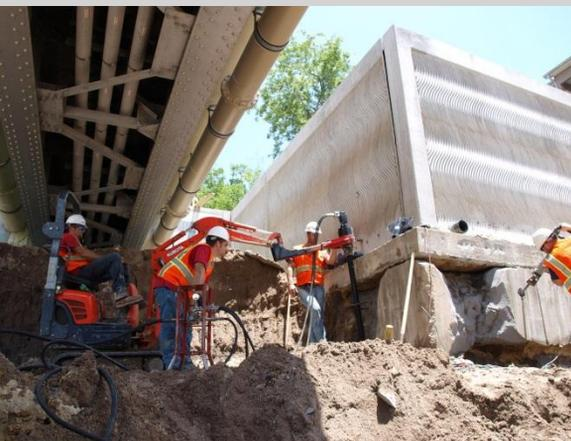
**Solution:** The immediate concern was to prevent the collapse of the structure. The contractor formed around the perimeter of the footing where it was undermined. Several yards of grout were pumped into the void space to reestablish a temporary bearing surface.
