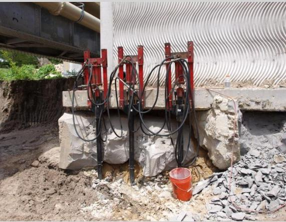
**Continue:** diameter helical piles to raise and stabilize the structure. The grout that was placed in the void space had to be partially removed at the pile placement locations in order to place the underpinning brackets and piles.
