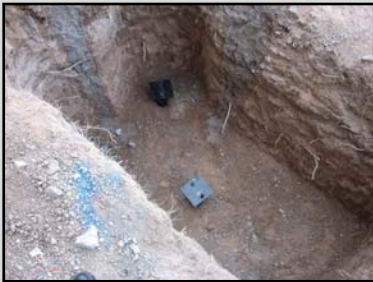
Pile cap ready for reinforcement and concrete
