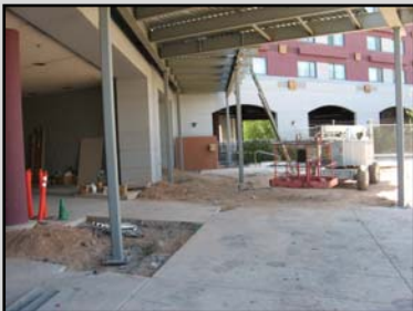
Columns installed on pile caps
