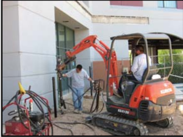
Driving helical pile
