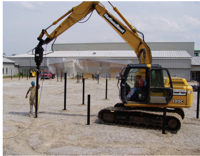
FIGURE 3-25 : Installation of New Construction Piles
