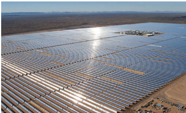
FIGURE 1-5 : Aerial Photo of Solana Solar Field (Taken On August 18, 2013)
