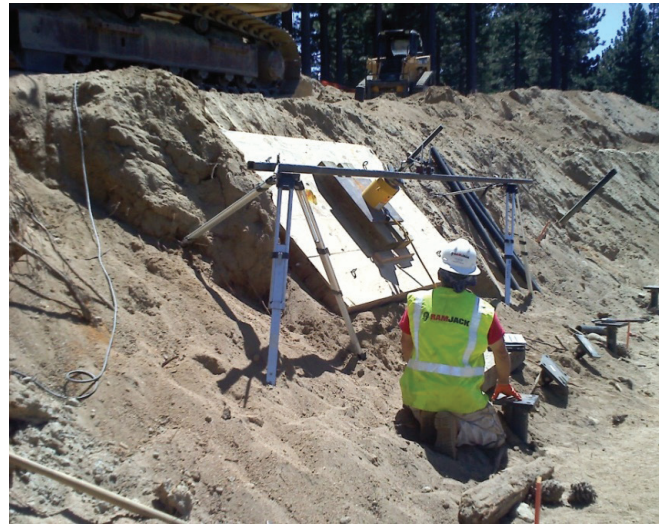
FIGURE 3-18 : Proof Load Test Setup on Helical Tieback Anchor
