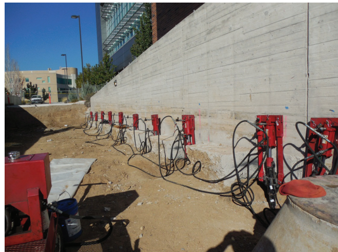
FIGURE 5-9 : Ram Jack Multi-Lift System
