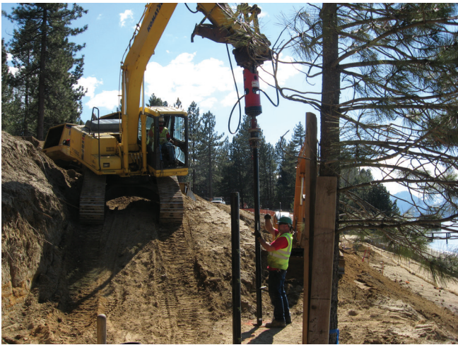
FIGURE 3-24 : Track Hoe Used to Install 5 5/8 in. [143 mm] Helical Piles
