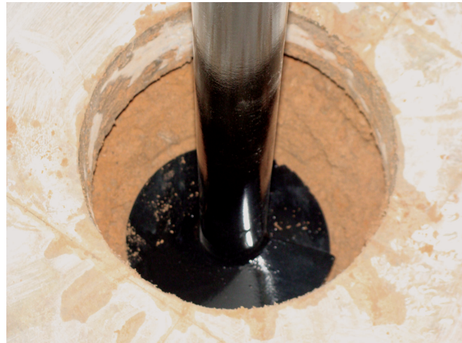
FIGURE 3-27 : Helical Installation Through Concrete Floor Slab
