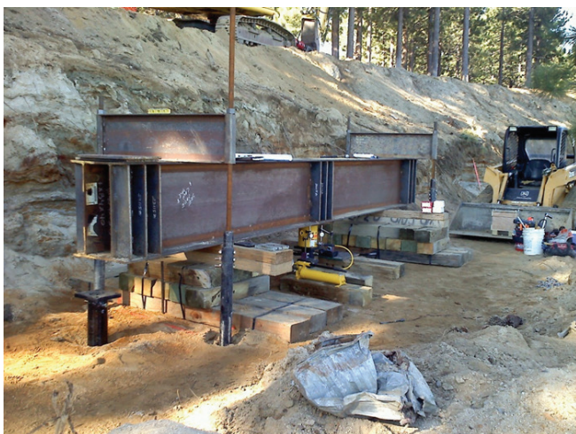
FIGURE 3-16 : Pile Load Compression Test Setup
