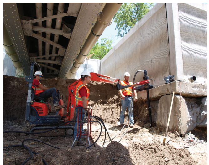
(b) Mini-Excavator Used for Installation
