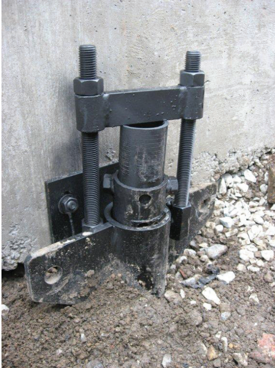
FIGURE 5-7 : Installed Driven Pile with Support Strap Assembly
