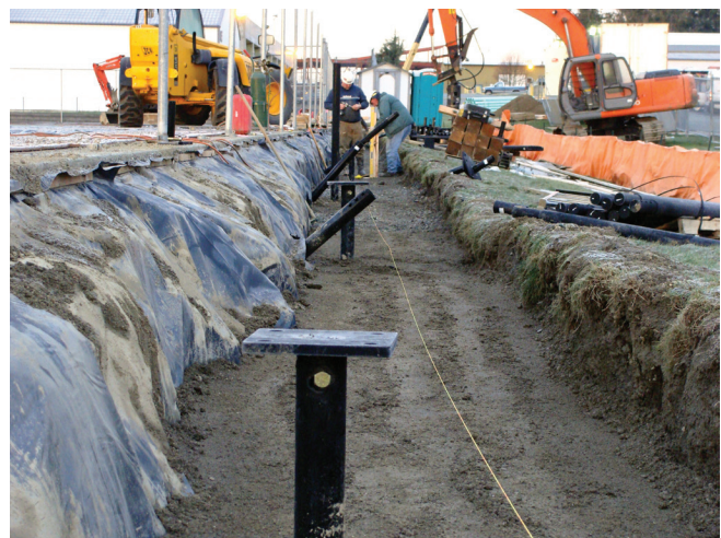
FIGURE 3-3 : New Construction Bracket
